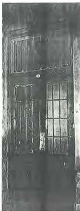
32 Doorway of the Budapest Clinic, Apt. no. 5 at 12 Mészáros Street (Judith Dupont)
